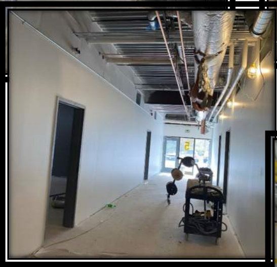
Prime & 1 st Coat Paint November 11, 2021
