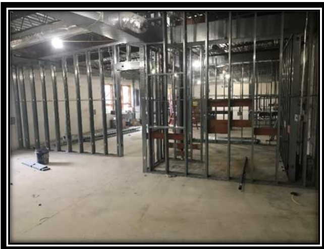
Area C Framing and In-Wall Rough-In March 18 th , 2021
