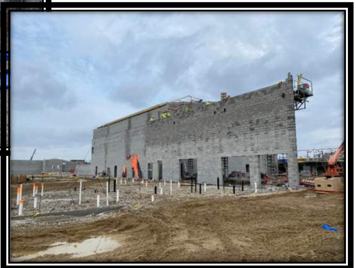
Area C Interior Masonry Bearing Walls February 18, 2020
